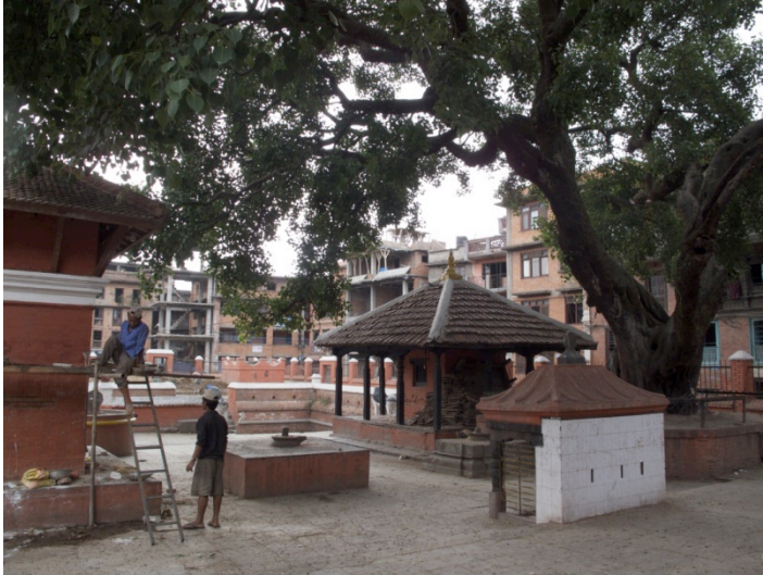
Figure 12: Kunbheshwar temple at Patan
